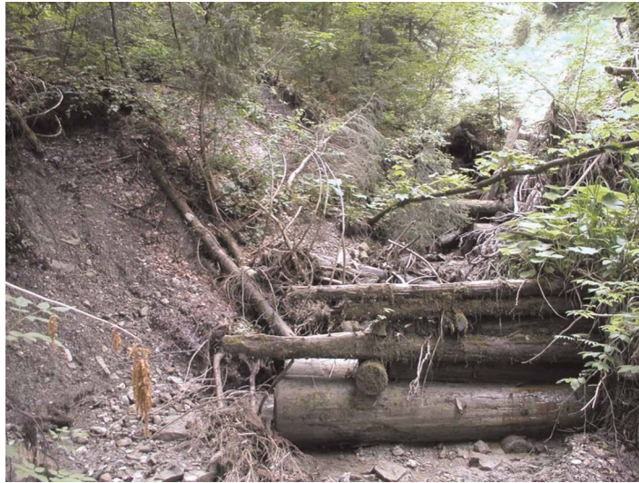
Fig. 6. Just one of thousands of torrent control structures that require maintenance.
